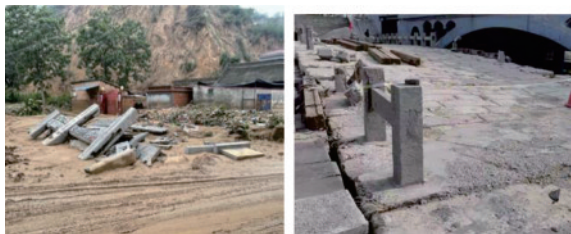
(a) 巩义孟氏石坊被洪水冲毁 (b) 鹤壁汤和桥栏杆望柱断裂缺失
